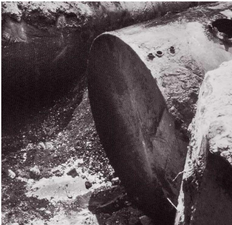
This tank excavation reveals a pool of leaked oil soaking into the ground.
