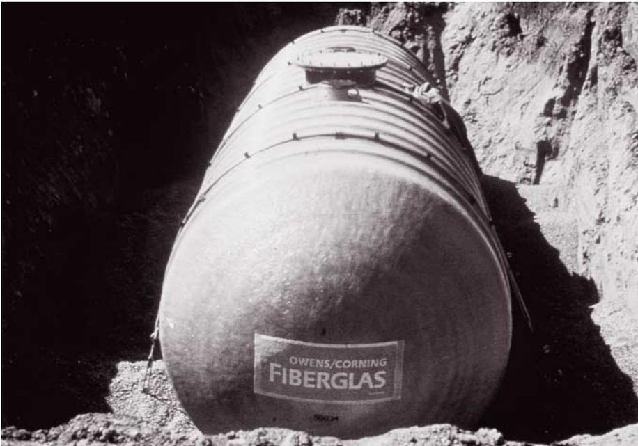
New installation of a fiberglass underground tank.
