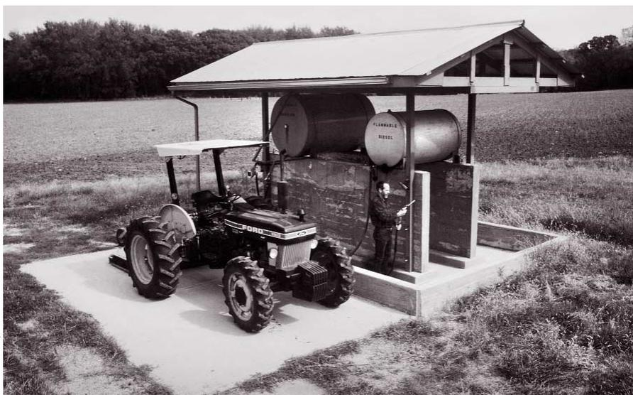
These above-ground tanks have a concrete pad and dike to contain spills and overfills.
